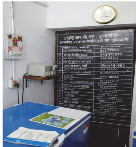
Picture 8. Placement of voltage stabilizer
